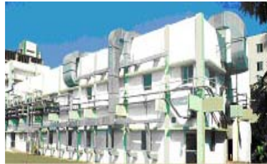
Sucrolose Manufacturing Facility
